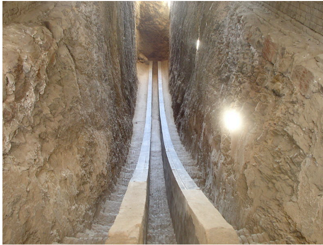
Figure 3: Ulugh Beg's observatory, Samarkand. His 36-meter radius sextant, dating from 1428, was sited in a circular arc between these marble walls (courtesy Alex Ostrovski).
