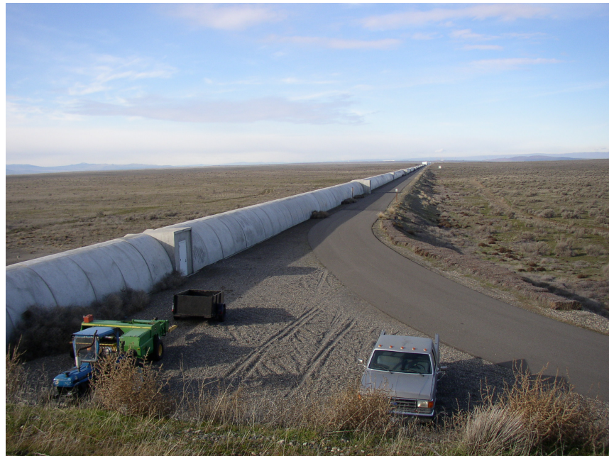
h / The part of the LIGO gravity wave detector at Hanford Nuclear Reservation, near Richland, Washington. The other half of the detector is in Louisiana.
