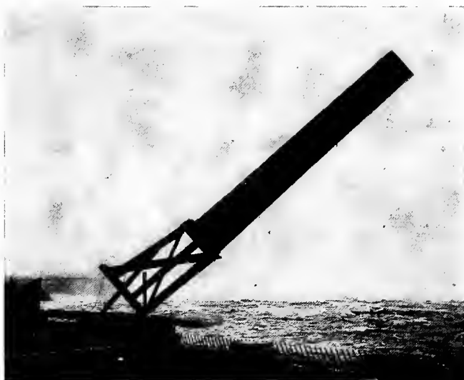
Fig. 78. Concrete dam falling into place, Niagara, N. Y.
