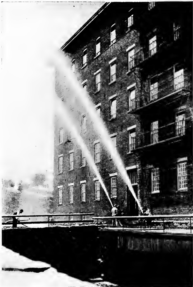
Force illustrated by two fire streams being delivered by the pump service of the large cotton mills of B.B. & R. Knight at Natick, Rhode Island. One stream is being held by men in correct position, the other by men who have been crowded into an awkward and dangerous position. Pressure shown on the gauge at the hydrant was 75 pounds per square inch.
