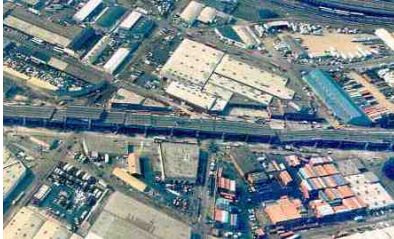
1 / The collapsed section of the Nimitz Freeway
