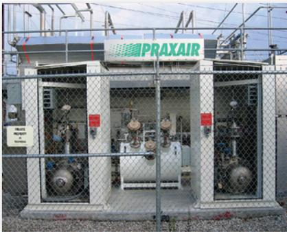
*Two 1kW pulse tube cryocoolers installed at HTS cable site
