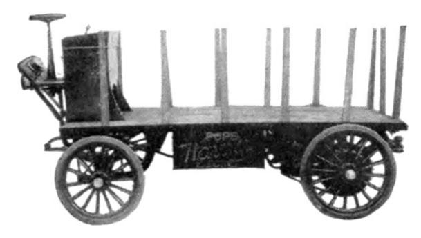
BODY: Stake platform CAPACITY: One ton WHEEL-BASE: 92 inches
