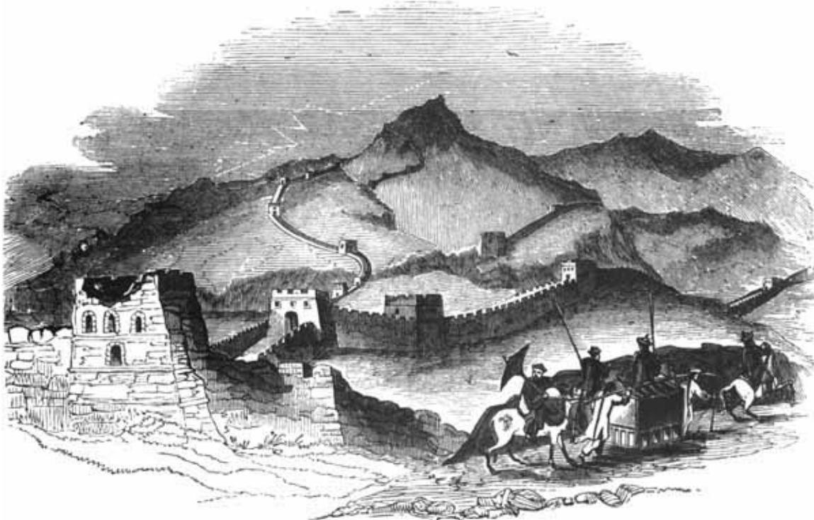
THE GREAT WALL OF CHINA.
