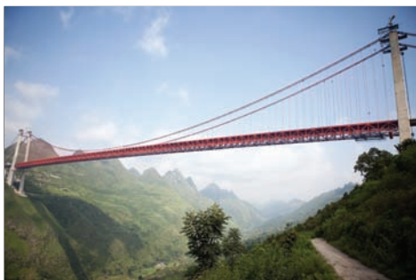
Recently completed Baling River Bridge in China's Guizhou province (2.25 km long and soaring 400 m above the Baling River). The tension in its cables and forces on its towers are described using vectors.
