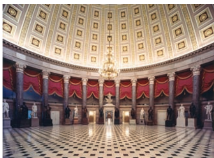
FIGURE 18 The ellipsoidal dome of the National Statuary in the U.S. Capitol Building creates a “whisper chamber.” Legend has it that John Quincy Adams would locate at one focus in order to eavesdrop on conversations taking place at the other focus.
