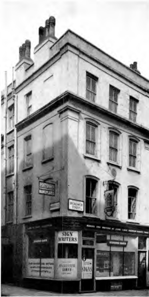
Blake's first house, No. 28 Broad Street, where God appeared in an upstairs window.
