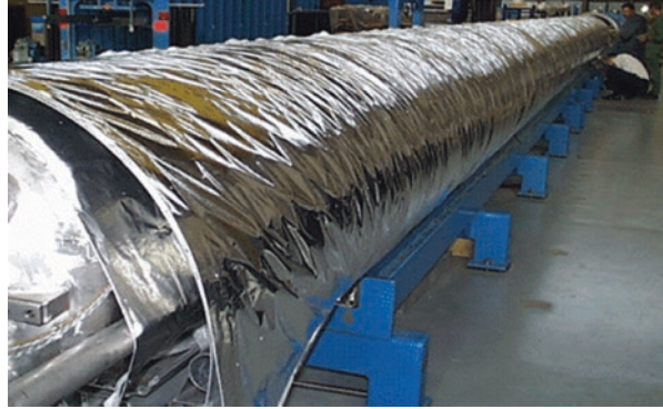
Fig. 2.12 Prefabricated MLI blankets are being installed around an accelerator superconducting magnet
