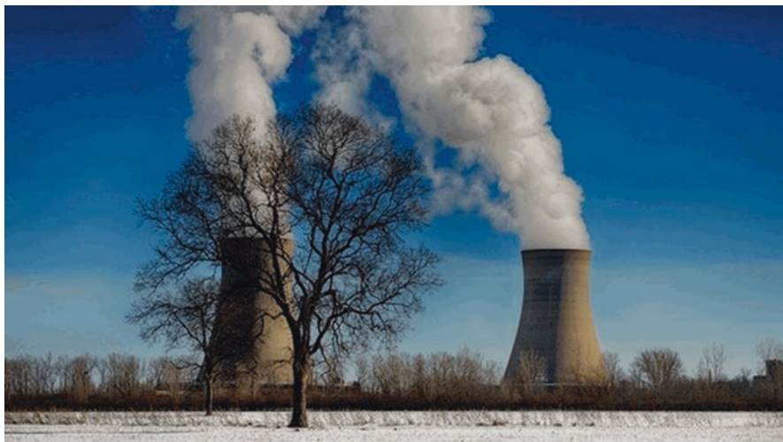
Fig. 1.20 A nuclear power plant south of Detroit, Michigan
