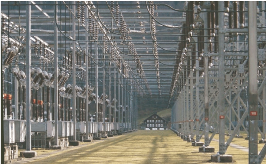
Fig. 3.2 Illustration of smart grid transmission (Courtesy of Siemens Corporation)
