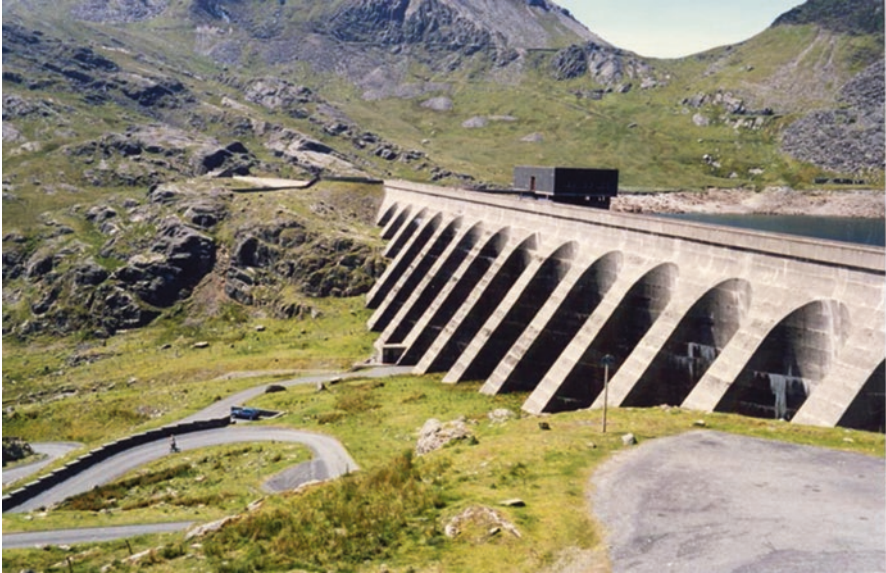
Fig. 8.10 Llyn Stwlan dam of the Ffestiniog pumped storage scheme in Wales
