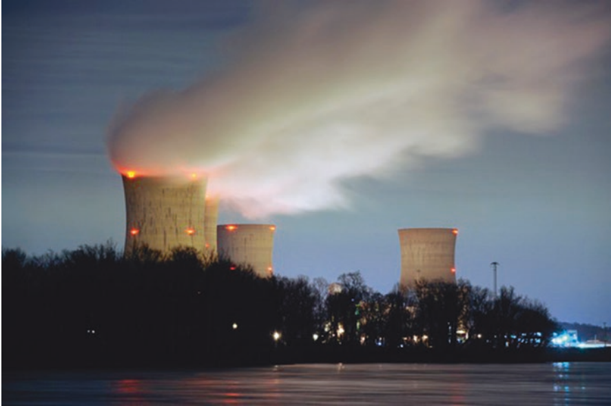
Fig. 1.23 Three Mile Island nuclear power plant at night in 2011 (Courtesy of REUTERS/Jonathan Ernst)
