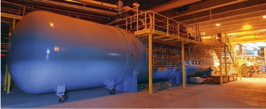
Fig. 2.22 Image of a 4.5 K cold box for the LHC (Linde) at CERN
