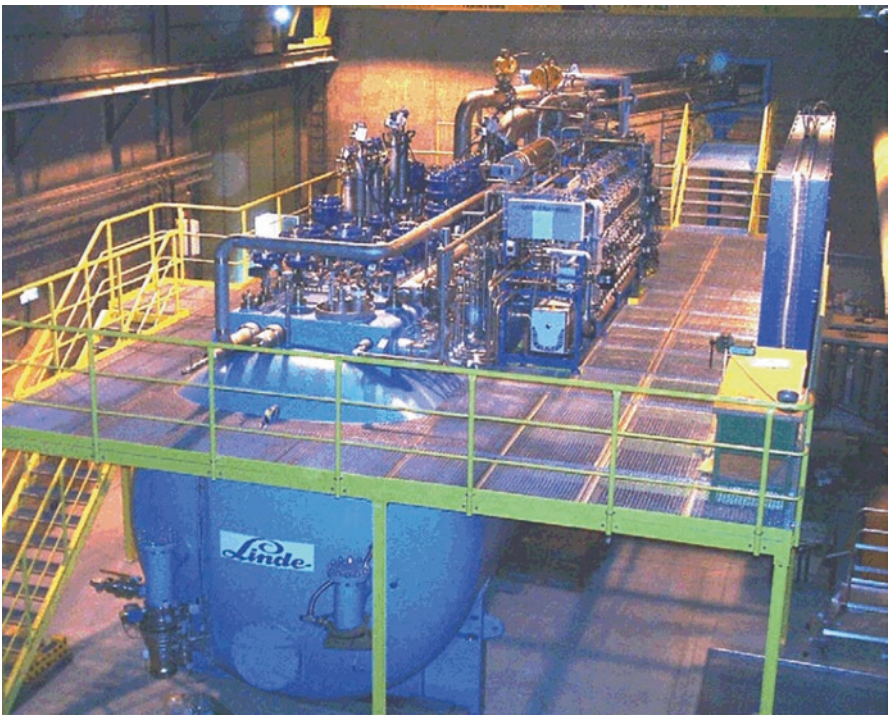
Fig. 2.23 Front view of 4.5 K cold box for the LHC (Linde) at CERN
