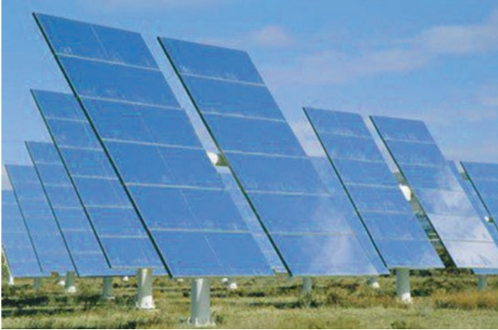
Fig. 4.18 Solar power panels (photovoltaic)
