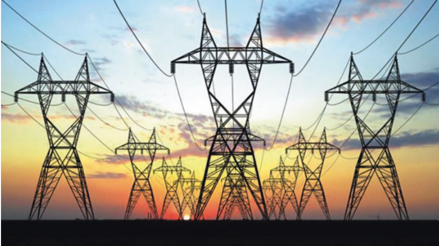
Fig. 3.1 High-power and high-voltage electricity tower distribution grids
