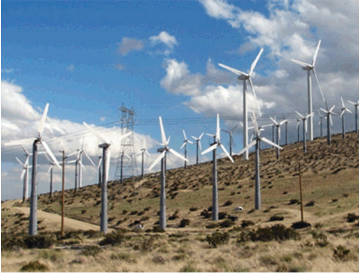
Fig. 4.17 Wind power farm
