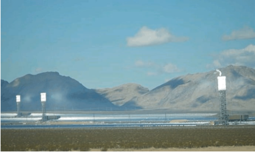
Fig. 4.6 The Ivanpah Solar Power Facility in California
