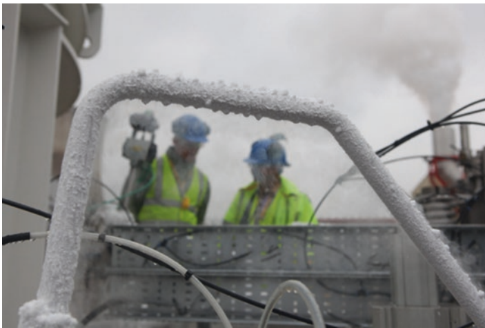
Fig. 3.4 Liquid air reheat and expansion to gas (Courtesy of Highview Power Storage)
