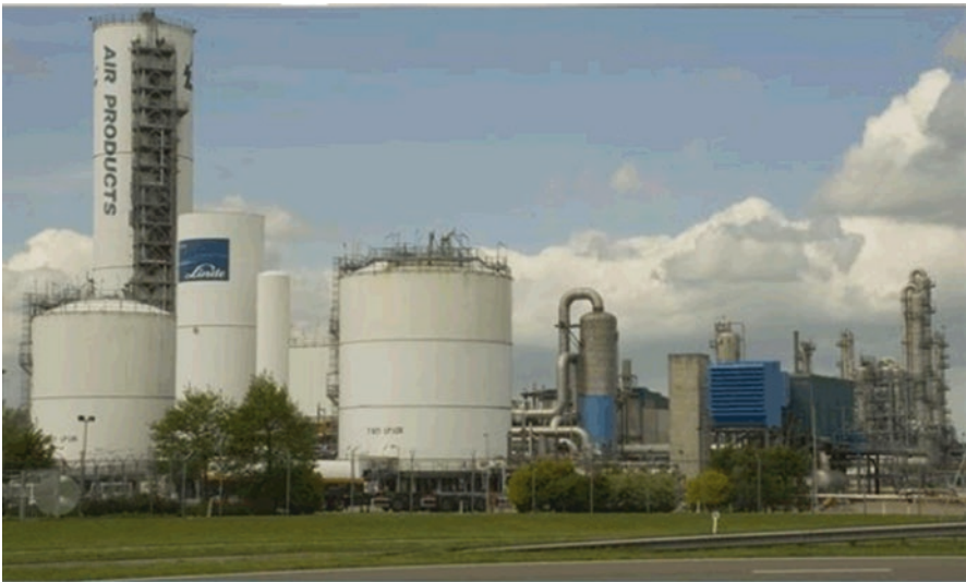
Fig. 2.2 Cryogenic air separation plant with heat exchanger and distillation column towers
