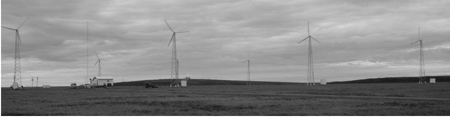
FIGURE 9.18 Wind turbines for diesel fuel saving at Kotzebue, Alaska. In the photo are seven Atlantic Orient wind turbines, 50 kW.
