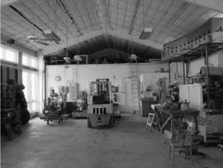
FIGURE 8.9 Interior of workroom showing that electrical lights are not needed due to daylighting.
