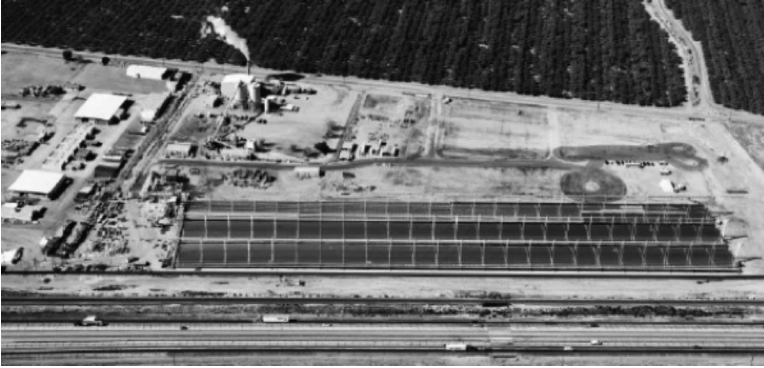
FIGURE 7.10 Linear Fresnel reflector, Kimberlina plant, 5 MW. (Courtesy of Ausra.)
