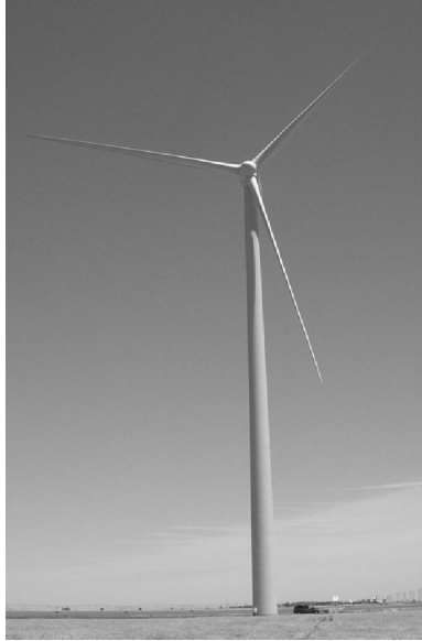
FIGURE 9.14 Vestas V90 3-MW wind turbine. Notice minivan next to the tower.
