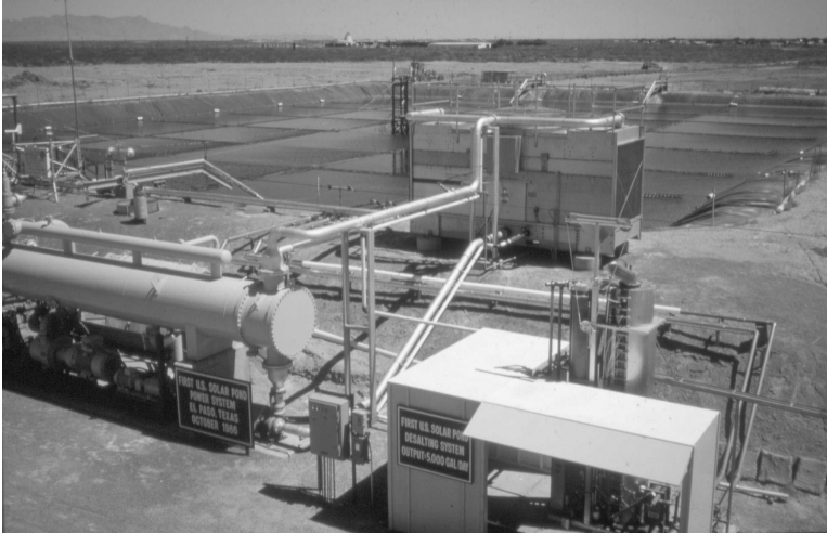
FIGURE 7.20 El Paso solar pond with Rankine-cycle engine (100 kW) for electric generation in the foreground.
