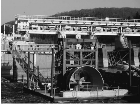
FIGURE 12.12 In-river system, 250 kW, on Mississippi River, Hastings, Minnesota. (Courtesy of Hydro Green.)
