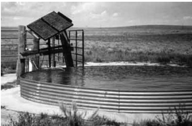
FIGURE 6.22 PV with passive tracker for pumping water for livestock. (From National Center for Photovoltaics, National Renewable Energy Laboratory (NREL), http://www.nrel.gov/ncpv .)
