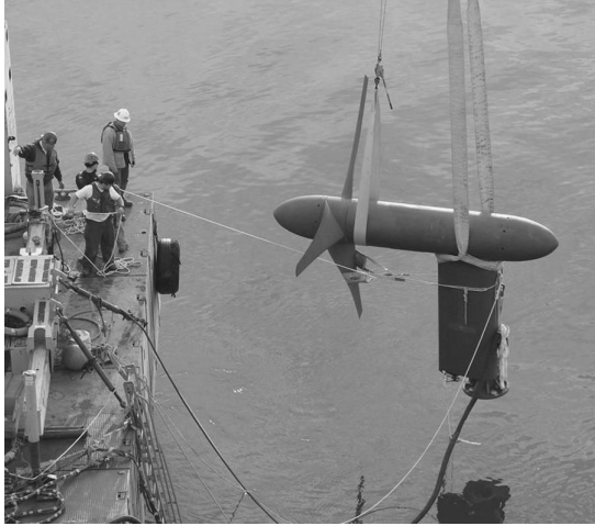
FIGURE 12.15 Tidal turbine, 35 kW, being installed in East River, New York City. (Courtesy of Verdant Power.)
