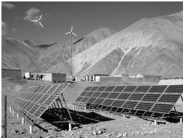
FIGURE 9.17 China village power system (PV/wind/diesel), 54 kW. (Courtesy of Charlie Dou.)
