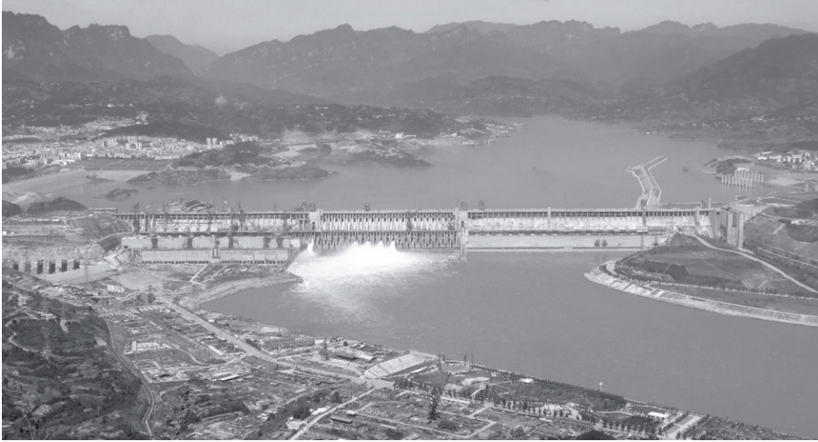
FIGURE 12.3 Three Gorges Dam, 22.5 GW, on the Yangtze River, China. (Courtesy of HydroChina.)
