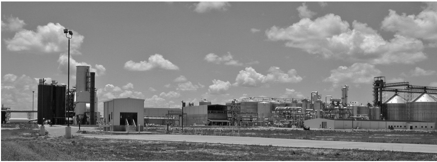
FIGURE 10.14 Ethanol plant near Herford, Texas.
