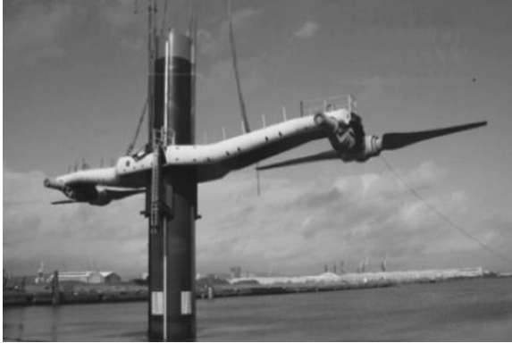
FIGURE 12.16 Tidal system, 1.2 MW, in Strangford Narrows, Northern Ireland. (Courtesy of Sea Generation).
