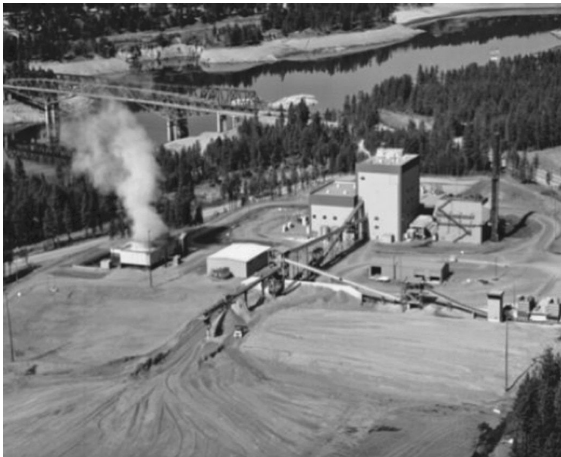
FIGURE 10.6 Power plant fueled by wood, Kettle Falls, Washington. (From NREL, http://www.nrel.gov/biomass .)
