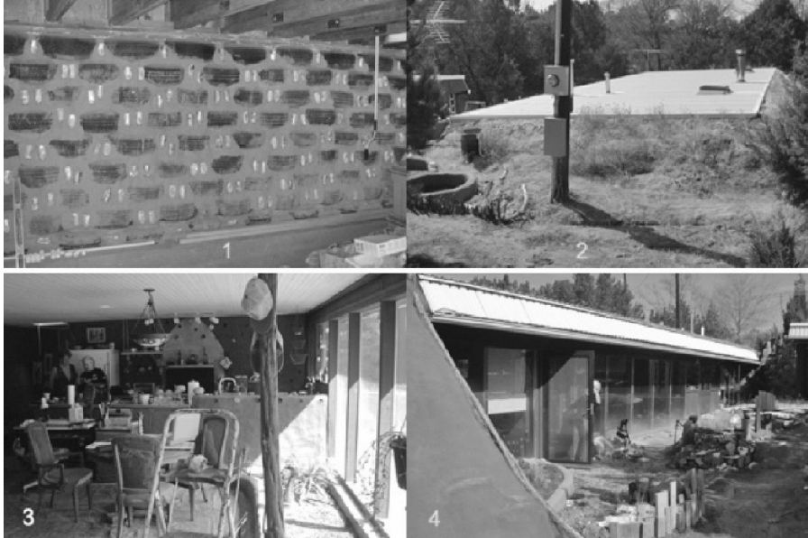
FIGURE 8.19 Zavatsky home, next to Camp Harrington on Ranch Road 1541 near Canyon, Texas. Passive solar home (17 by 6 m) and adjoining workshop (9 by 6 m). Both have tire walls and are bermed on three sides; roofs have R55 insulation and are designed for catching rainwater. (1) Unfinished tire wall in workshop. Notice cans for space filler. (2) Roof of home showing the berm; cistern catchment on left. (3) Interior of the home. (4) Exterior of home; notice overhang for shading during the summer. Photos taken March 27, 2004.
