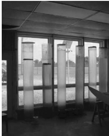
FIGURE 8.5 Water tubes for more thermal mass and added food color became stratified. Note water level due to evaporation because of poor cover. Lower sash on windows has manual opening.
