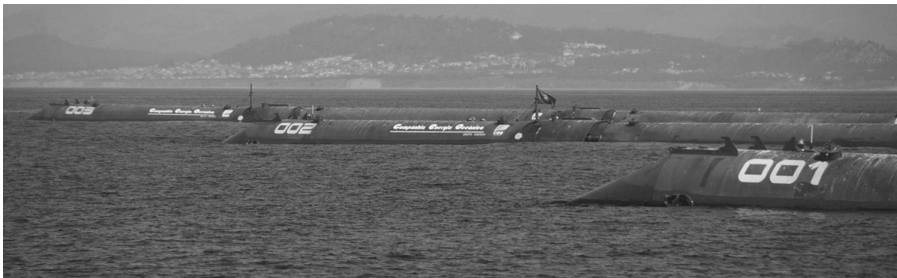
FIGURE 12.24 Installation of three units at Aguçadoura, Portugal, 2.25 MW total power. (Courtesy of Pelamis Wave Energy.)
