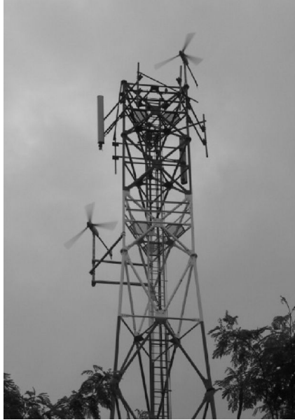
FIGURE 9.19 Two 1.5-kW wind turbines at telecommunication system, China. (Courtesy of Charlie Dou.)
