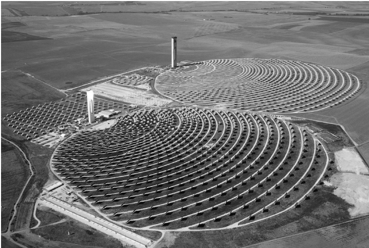
FIGURE 7.5 Abengoa power towers, Seville, Spain. Top is 11 MW, bottom is 20 MW. Notice that there are also PV panels. (Courtesy of Abengoa.)
