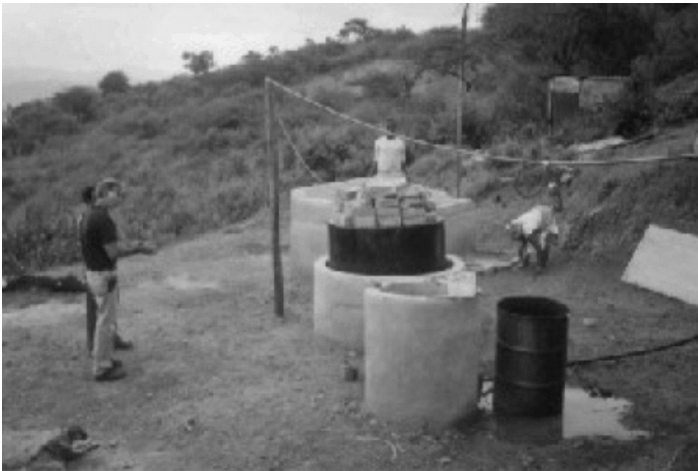
FIGURE 10.15 Floating roof biodigester in South Africa. (Courtesy of Solar Engineering, South Africa.)
