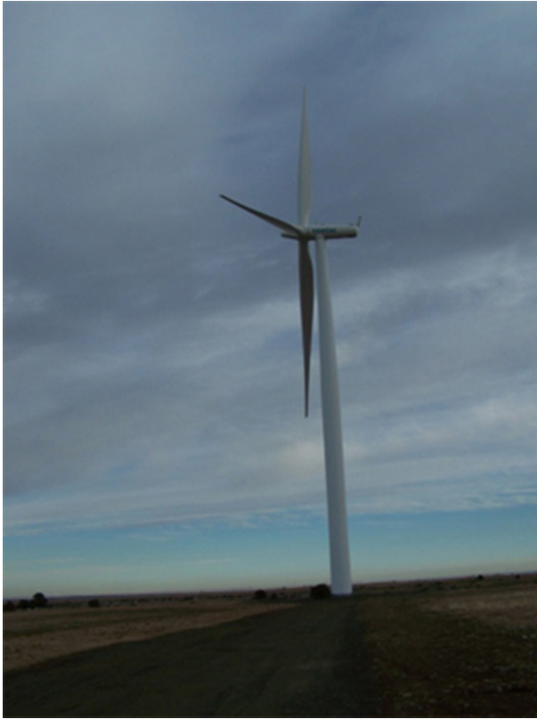
Figure 2.3. Wind turbine generator at National Wind Test Center. (Source: Courtesy of NREL.)
