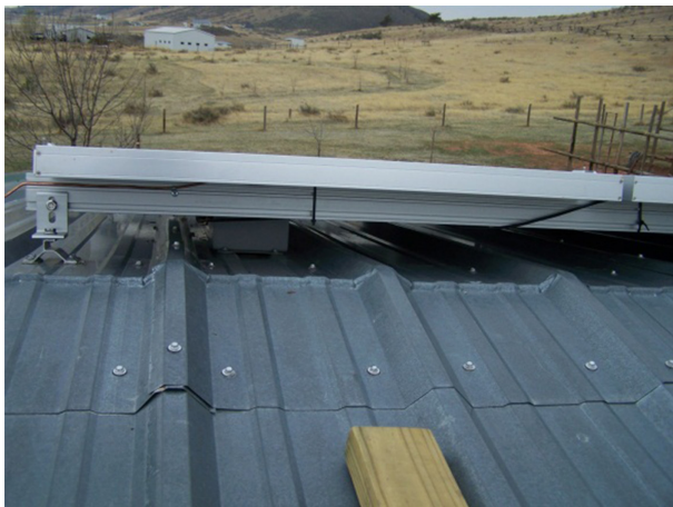
Figure 9.6. Roof-mount brackets.
